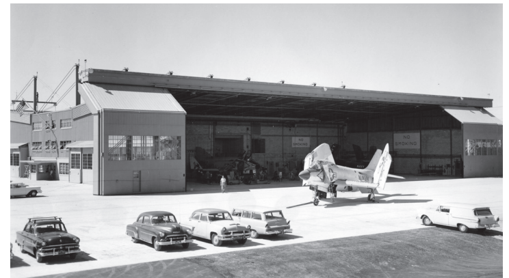
Flight Test Facility showing cable system for cantilever roof and large hanger doors, ca. 1959
