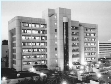
Murrah Federal Building in Oklahoma City prior to a vehicle bomb attack.
